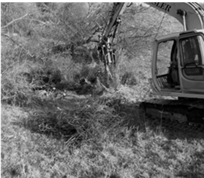
Fence wire and other debris being removed from a sinkhole in Monroe County, West Virginia. (Photo by Rocky Parsons)
