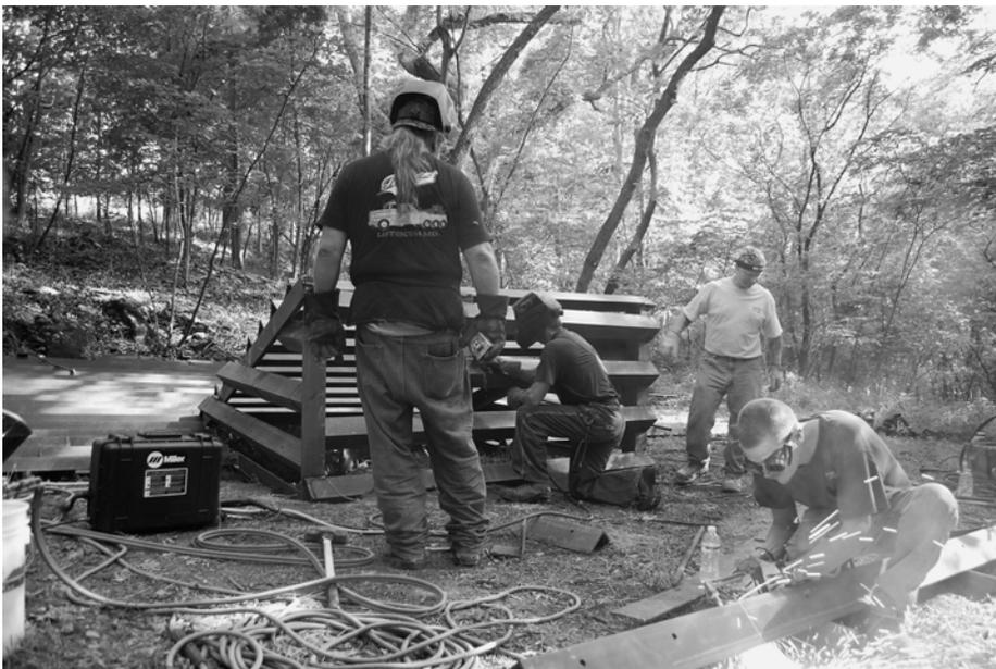
The welding crew working on the Front Royal Cave gate. The original gate was horizontal and difficult for bats to get through. The new steel structure provides an easier route for bats to get through. Photo by Nuch Songsasen.
