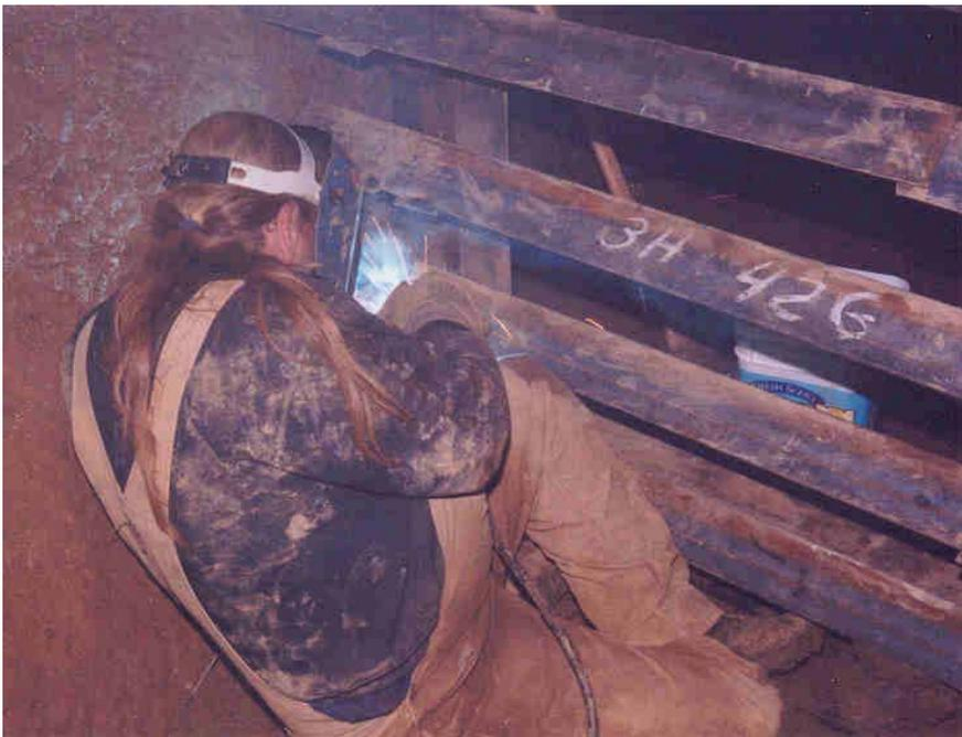
Craig Hindman, (also known as "Weldo") welding the gate together inside the cave. The longest horizontal rod is over 8 feet long and Craig used about 30 pounds of welding rod to assemble the gate. The spacing between the bars is carefully measured to allow bats to fly through but to stop humans.
